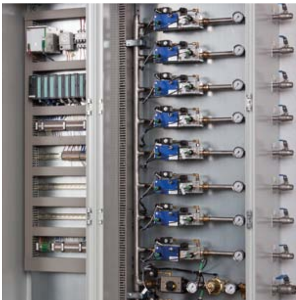
Gas dispensing system with mass flow controller
